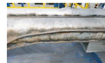
Pipeline maintenance (HTR)
